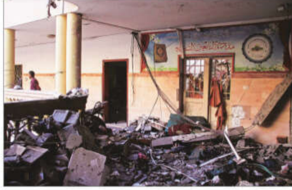
Damage at the site of an Israeli strike on a school sheltering displaced people in Gaza City on Saturday
